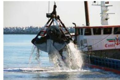
Dredging the lagoon to prepare for the installation of the flood barriers.
